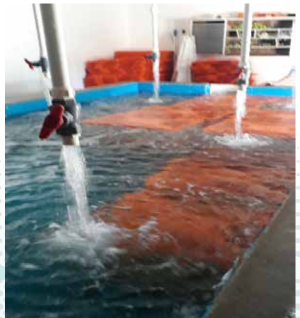
Figure 5 Holding tanks at Māhia depot—January 2019
