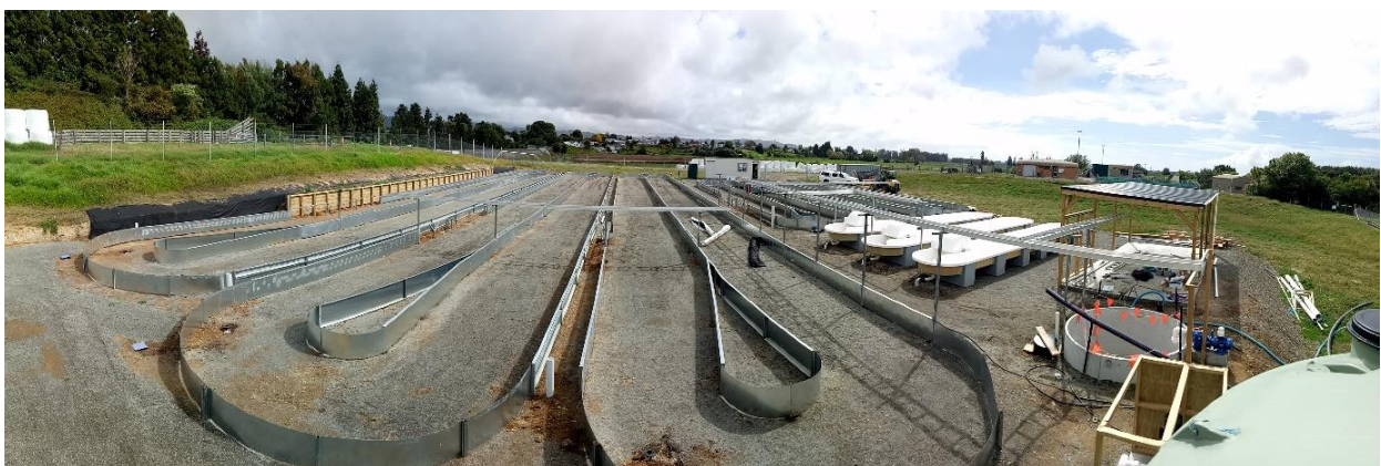
Figure A2. AquaCuro's freshwater algae bioremediation pilot plant under construction in Te Puke in collaboration with researchers at the University of Waikato (Photo: Chris Praeger/AquaCuro). The plant consists of 3 x 10 m high rate algal ponds (HRAPs), 3 x 25 m HRAPs and 3 x 50 m HRAPs. The 50 m long HRAPs are here yet to be lined with high density polyethylene liner.
